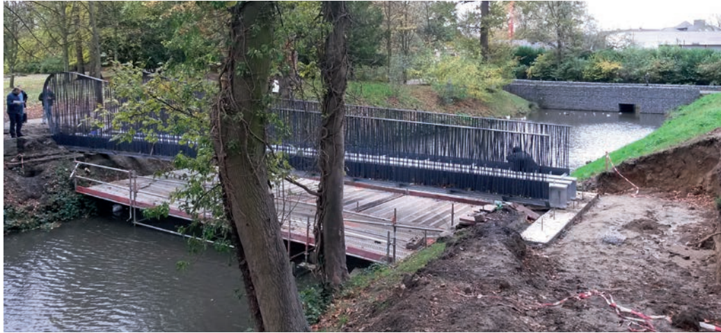
17 18 Construction of bridge two © Abscis Architekten
