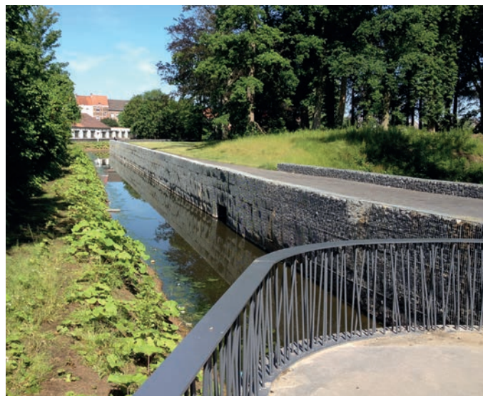
5 High-retaining wall in gabion © Abscis Architekten
