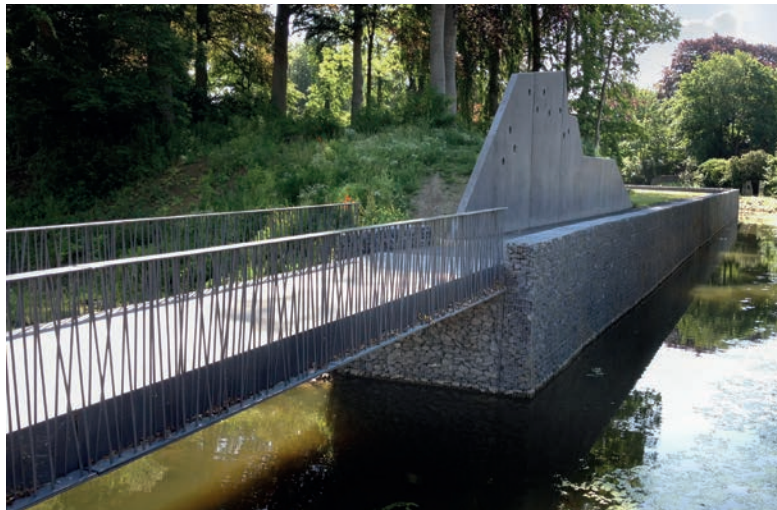
10 First bridge »with« gabion © Abscis Architekten
