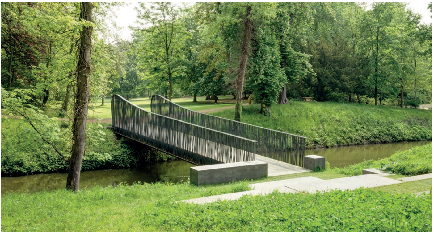
19 Concrete ornamental bridge after completion © Inge Claessens
